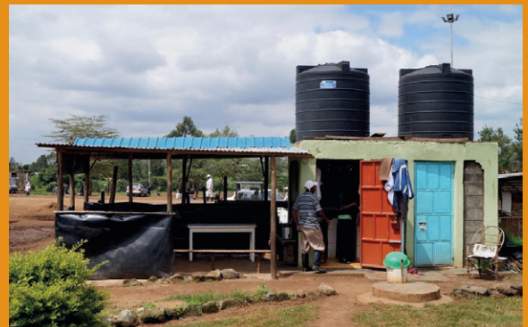
Biogas latrines at Dagoretti market, Nairobi.
