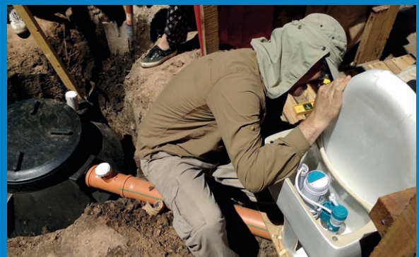
ERM Regional CEO for Latin America and the Caribbean, Carlos Pereyra, providing onsite support to install solar showers and toilets.
