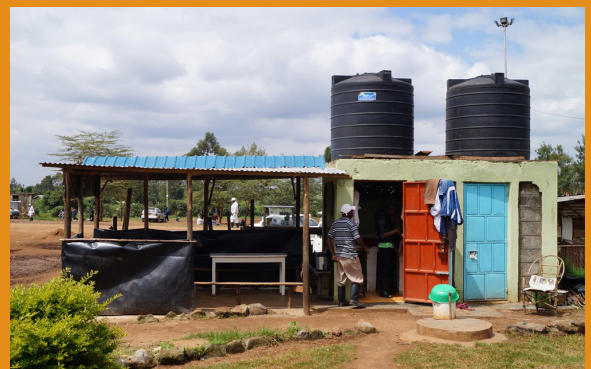
Biogas latrines at Dagoretti market, Nairobi.
