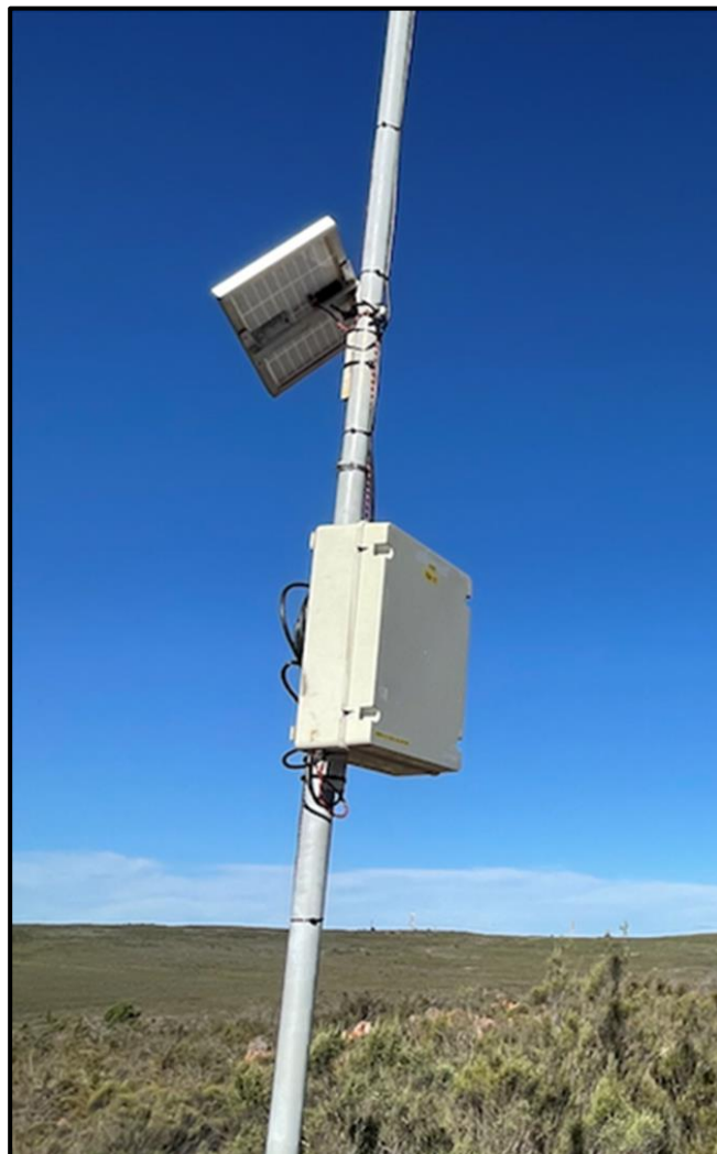
Figure 5: System on a 10 m mast at the proposed Hugo WEF
