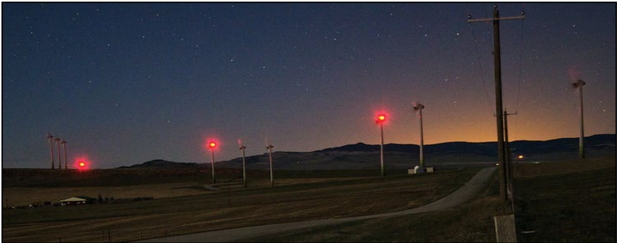
Figure 52: Aircraft warning lights fitted to the wind turbine hubs (Source: http://www.pinchercreekecho.com/2015/04/29/md-of-pincher-creek-takes-on-wind-turbine-lights )
