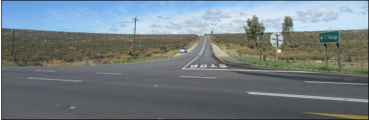
Photograph 3.1: Intersection of N1 and R318
