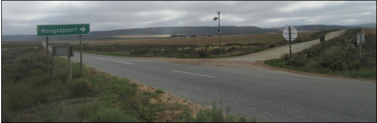
Photograph 3.3: Intersection of R318 and Nougaspoort road.
