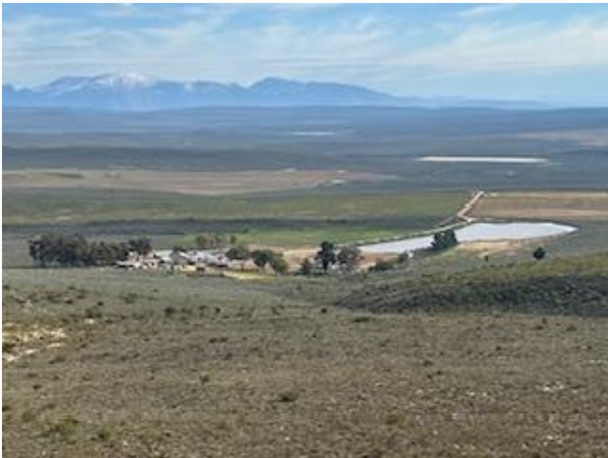
Photograph 3.18: Looking north from slopes of Waboomsberge, Kleinkraal yard (Farm 34) in middle ground, and a snow-capped Matroosberg in the distance. Some of the buildings on the yard are planned for conversion into tourist accommodation (Source: Karen Kritzing)
