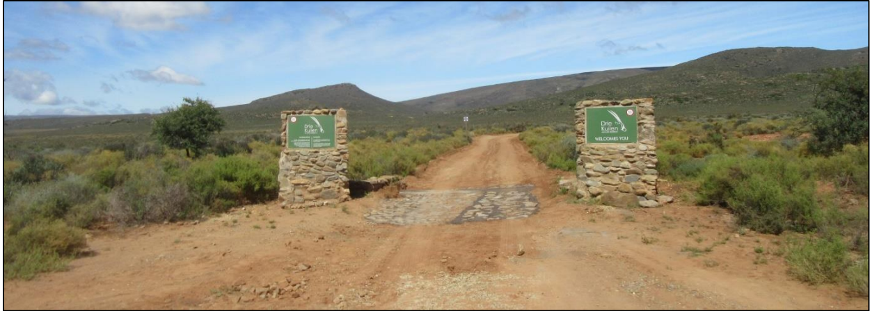
Photograph 3.16: Main entrance to Drie Kuilen Private Nature Reserve of the Nougaspoort Road
