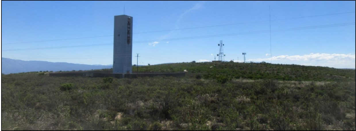
Photograph 3.3: Telecoms towers on Eendragt 38/1 at the crest of the Rooihoogte Pass, seen from the R318.
