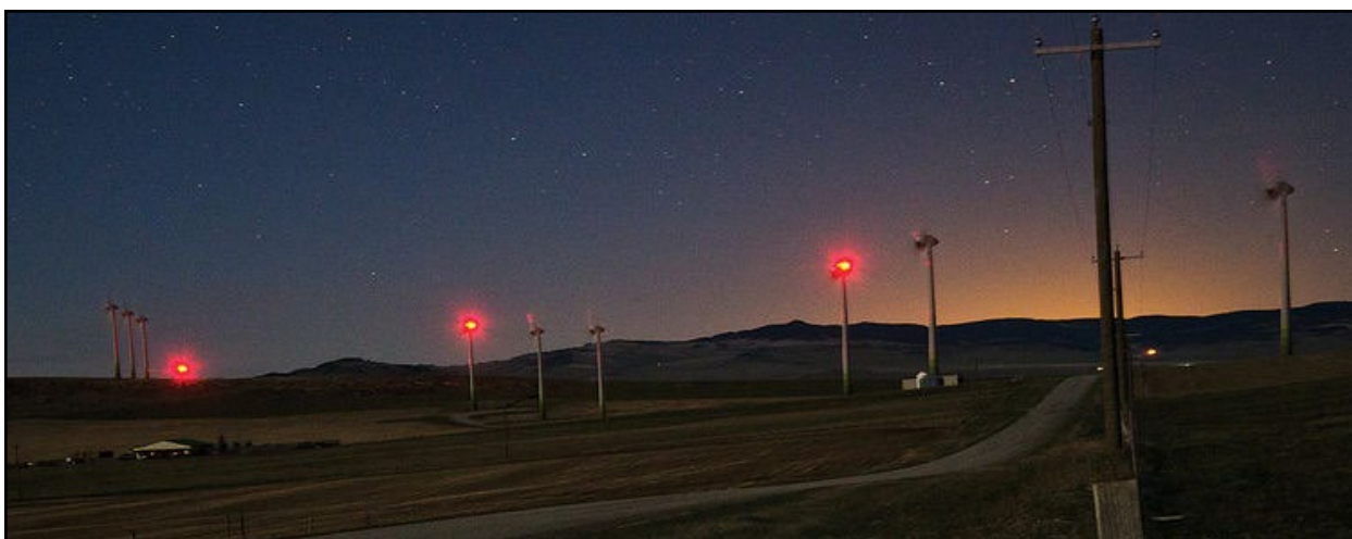
Figure 63: Aircraft warning lights fitted to the wind turbine hubs (Source: http://www.pinchercreekecho.com/2015/04/29/md-of-pincher-creek-takes-on-wind-turbine-lights )
