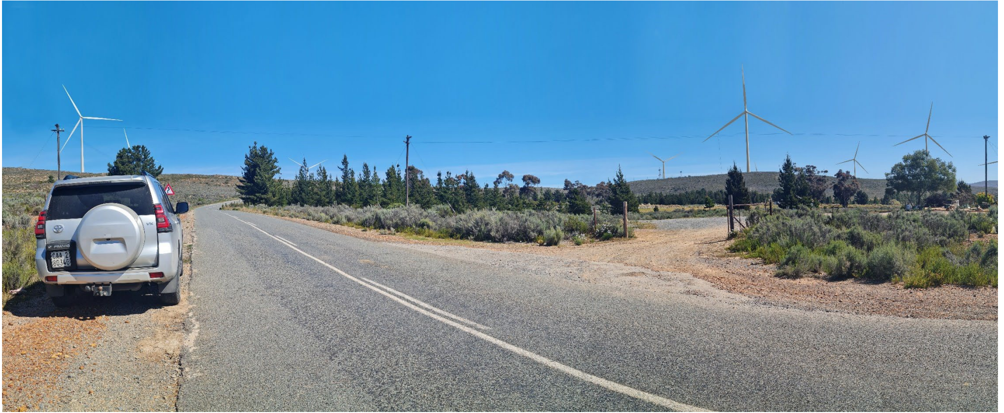
Figure 23: Photo simulation 4b- after. The closest wind turbine of the Khoe Wind Facility is 1 km from this point.
