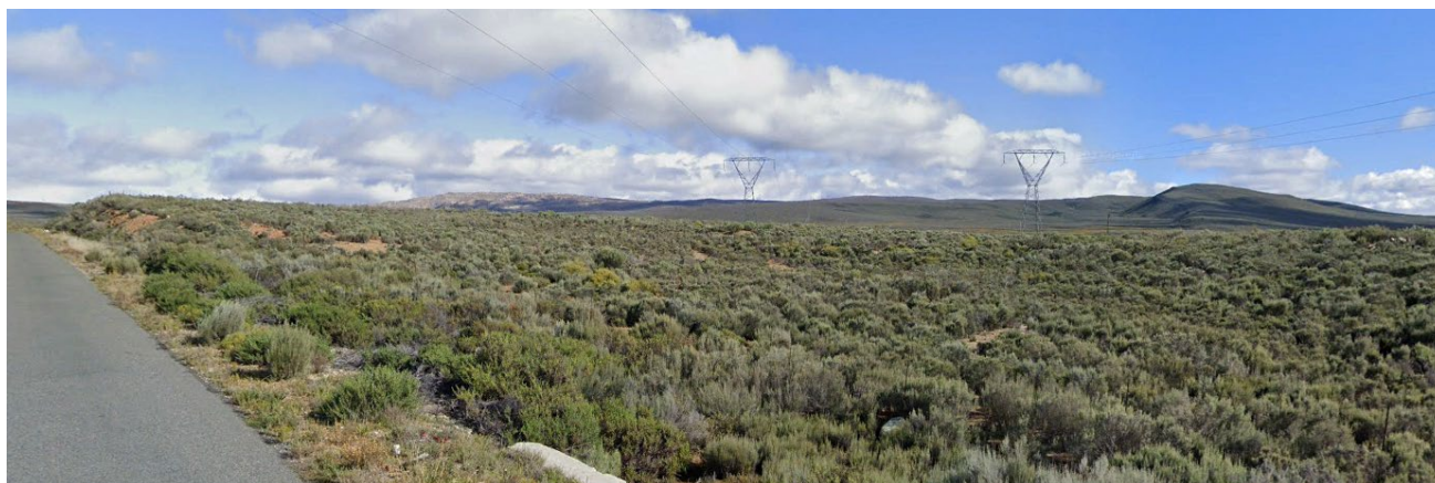
Figure 7: Existing power lines traversing the proposed Hugo site
